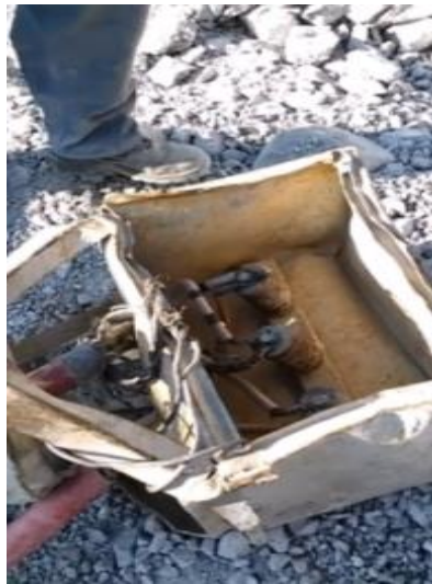
Figure 6. Example of intervention on corner transformers
